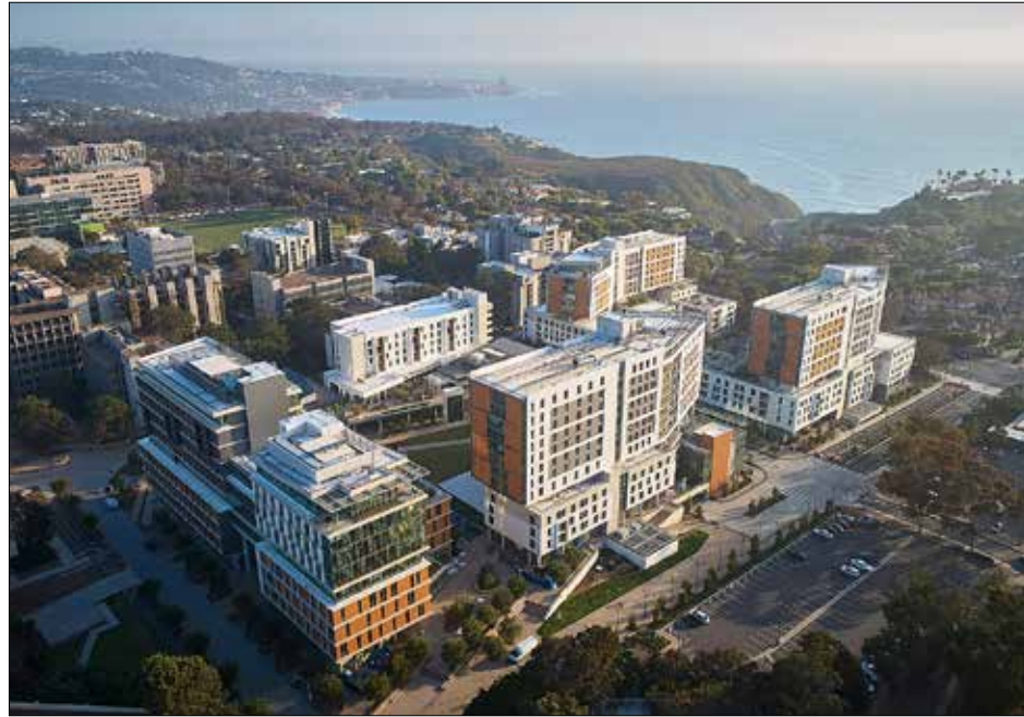
There's no lack of development at University of California San Diego. Shown here is the LEED Platinum Certified North Torrey Pines Living and Learning Neighborhood. Photo courtesy Tom Harris Photography
